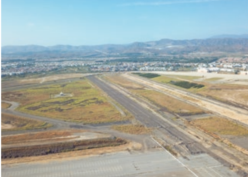
Proposed “Golf Course Site” for Irvine Veterans Cemetery in the foreground, with the ARDA site in the distance. PHOTO COURTESY OF THE CITY OF IRVINE
